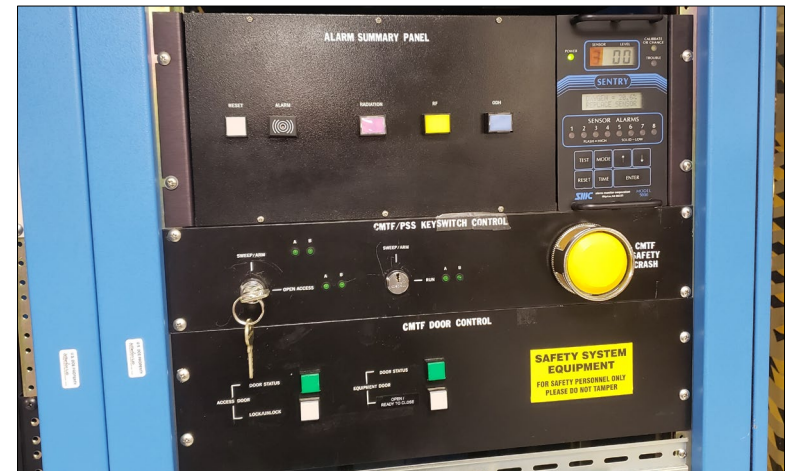
PSS Alarm Summary, key/door control, & ODH panels
