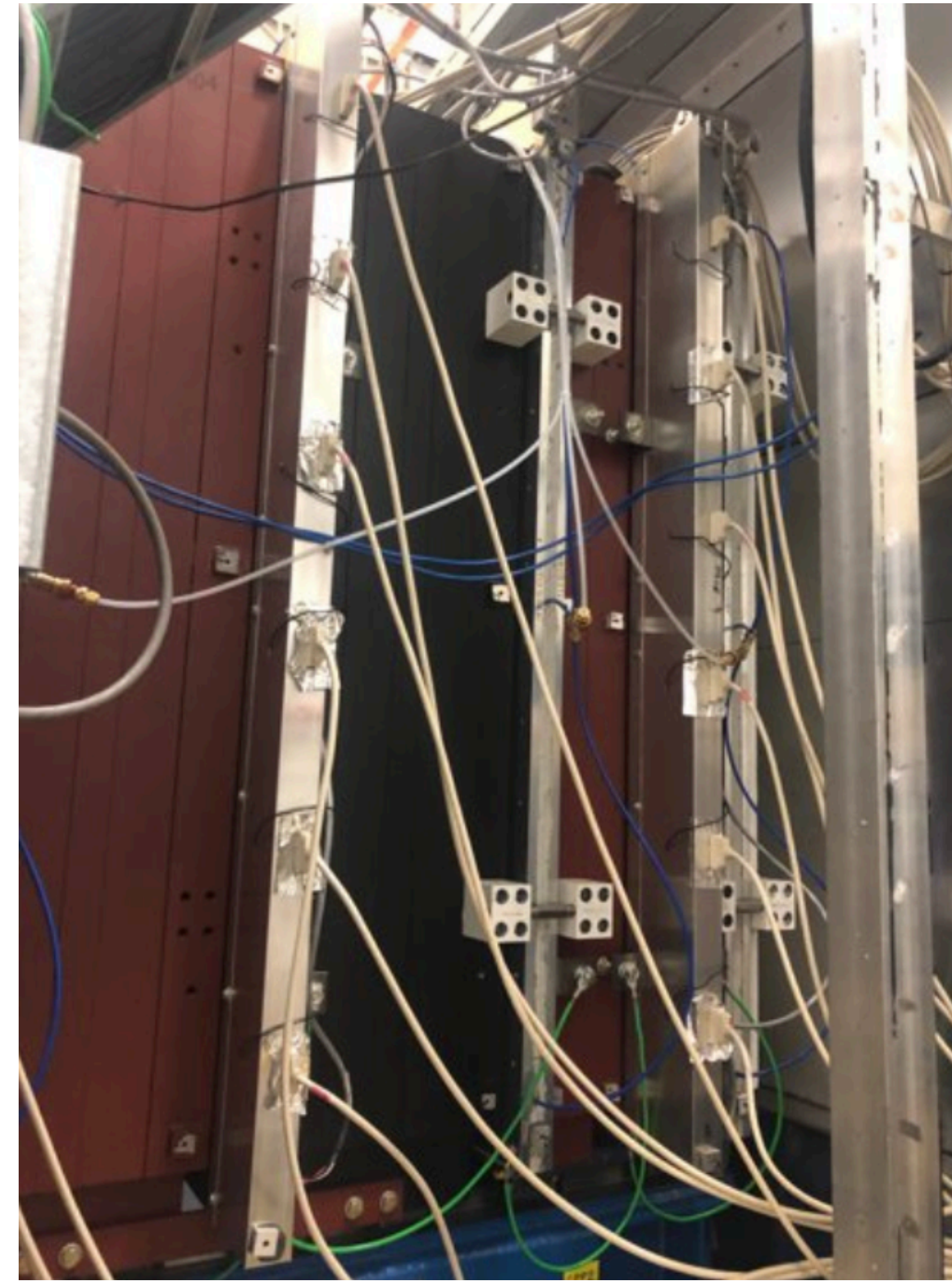
Chambers installed with Iron Absorbers
