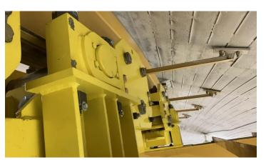
New trucks installed and the hanging supports were shimmed
