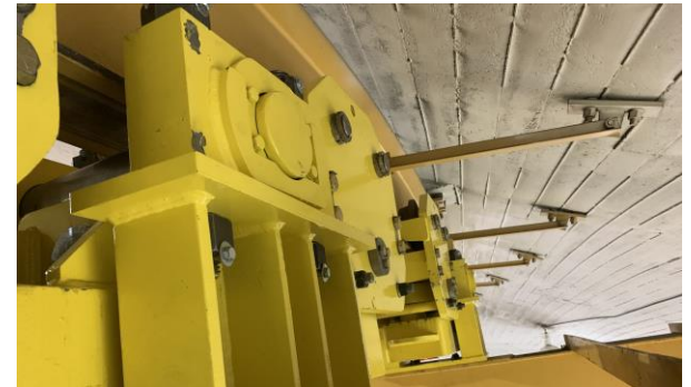
New trucks installed
