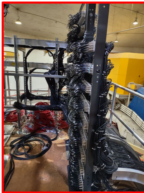
Cables from detector top to patch panel
