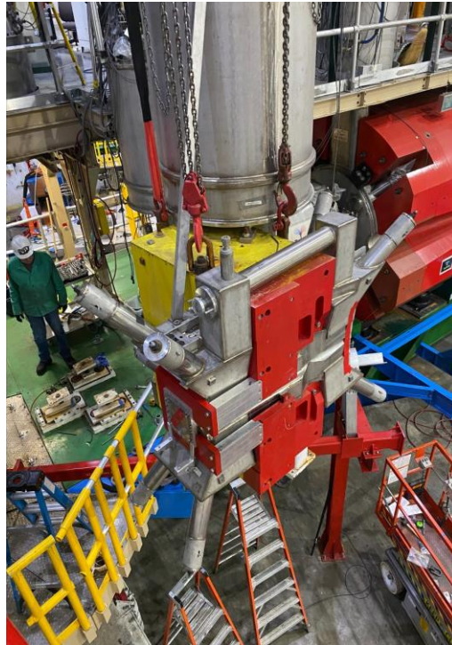
Removal of the SHMS HB magnet
