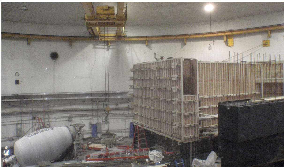
Vendor forming and pouring concrete for SHMS shielding house.
