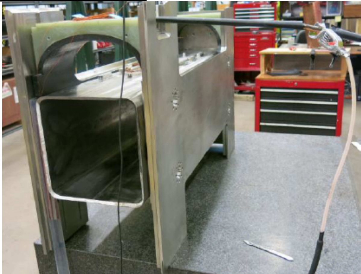
Top coil installed and undergoing hi-pot test.
