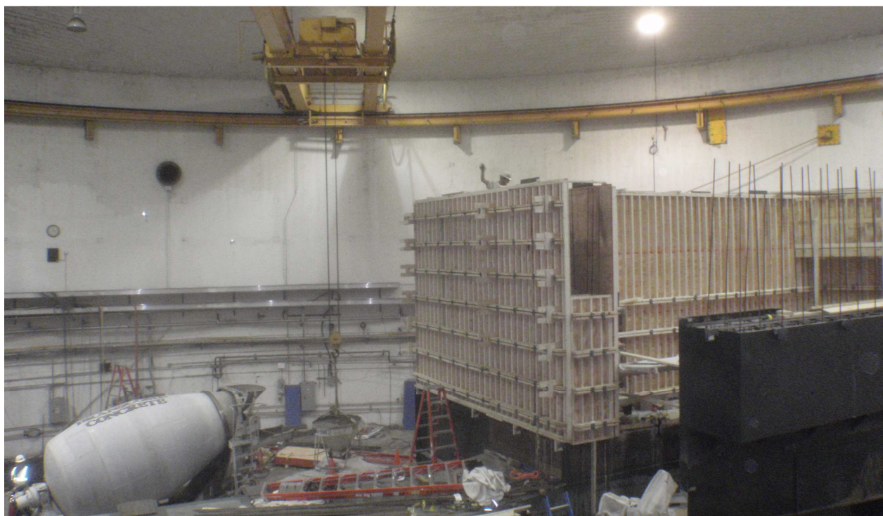
Forming placed for the concrete pour for the SHMS shield house.
