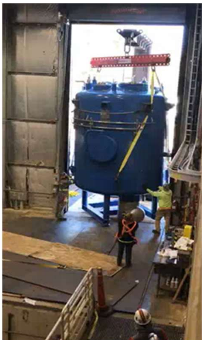
2K Cold Box moving into CHL
