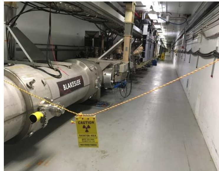
Radiation hazards due to activation
