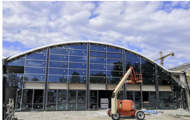
Figure 5. Front view of B5 during the renovation works.
