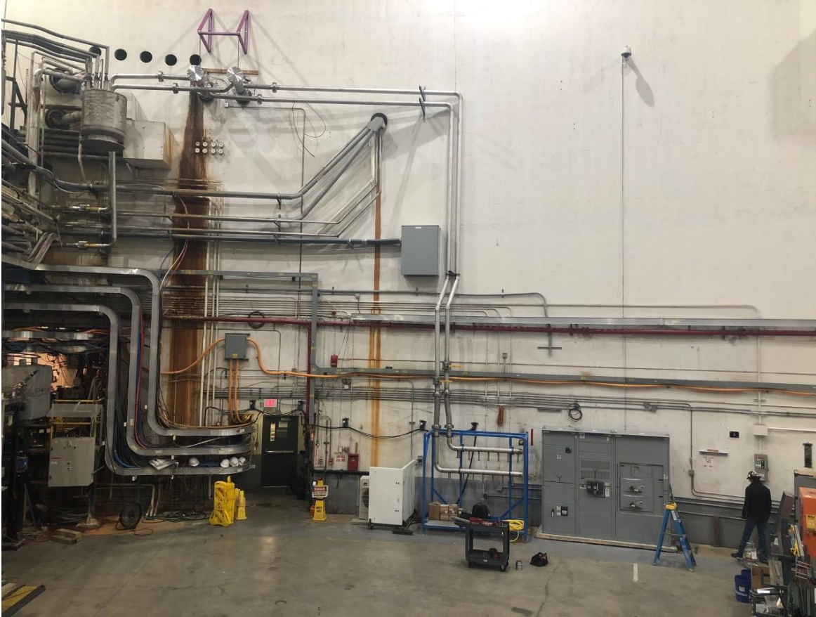
LCW Manifold & 2MVA Switchgear: In-Progress
