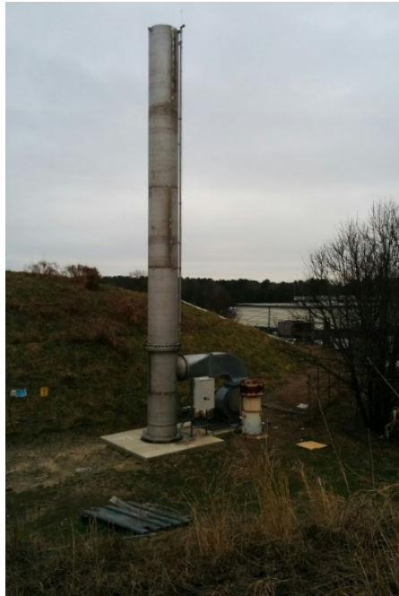
Target Exhaust System and Stack
