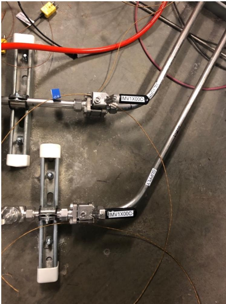
**Figure 10.** Dump LCW Supply & Return Valves
