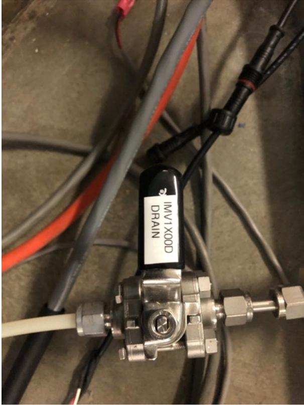
**Figure 12.** ¼" Nylon drain line
