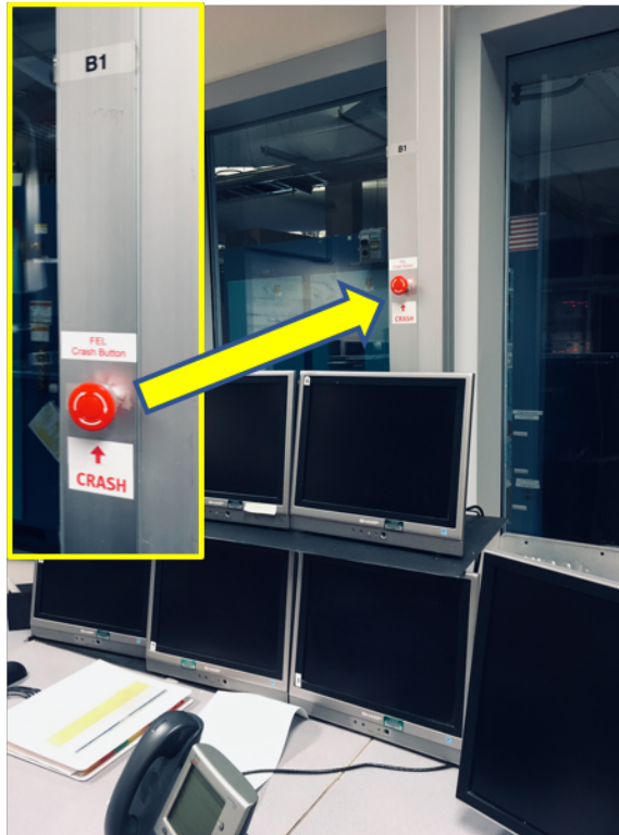
Figure 2. LERF Crash Button to be hit in case of emergency to shut off the equipment.
