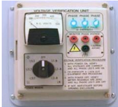
Figure 2 – VVU (Voltage Verification Unit)
