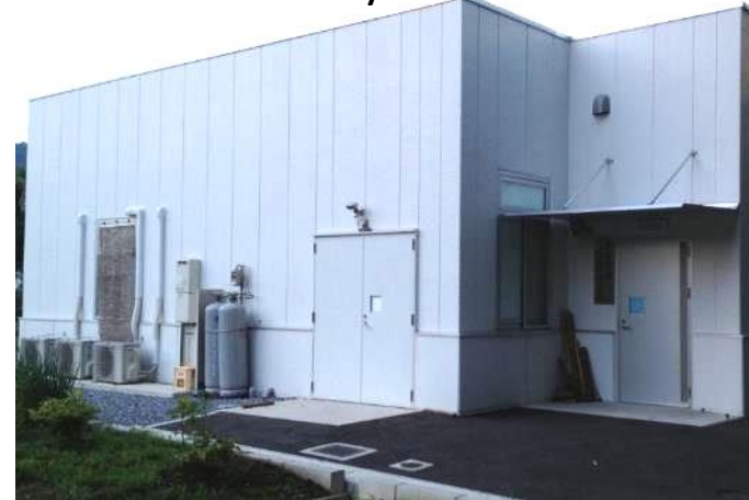
2012- Emulsion facility in Gifu-Univ.
