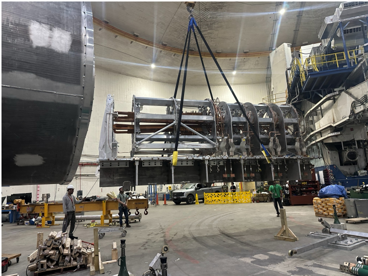
MOLLER toroidal magnets on beam line
