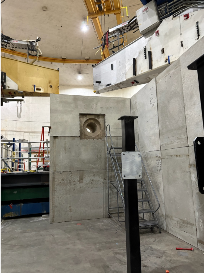
Target region shielding – partially installed
