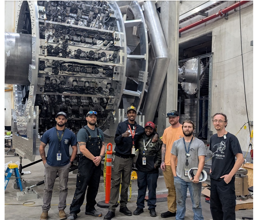
MOLLER Main detector segments were all installed in June. Shower Max detectors were all installed at end of September.
