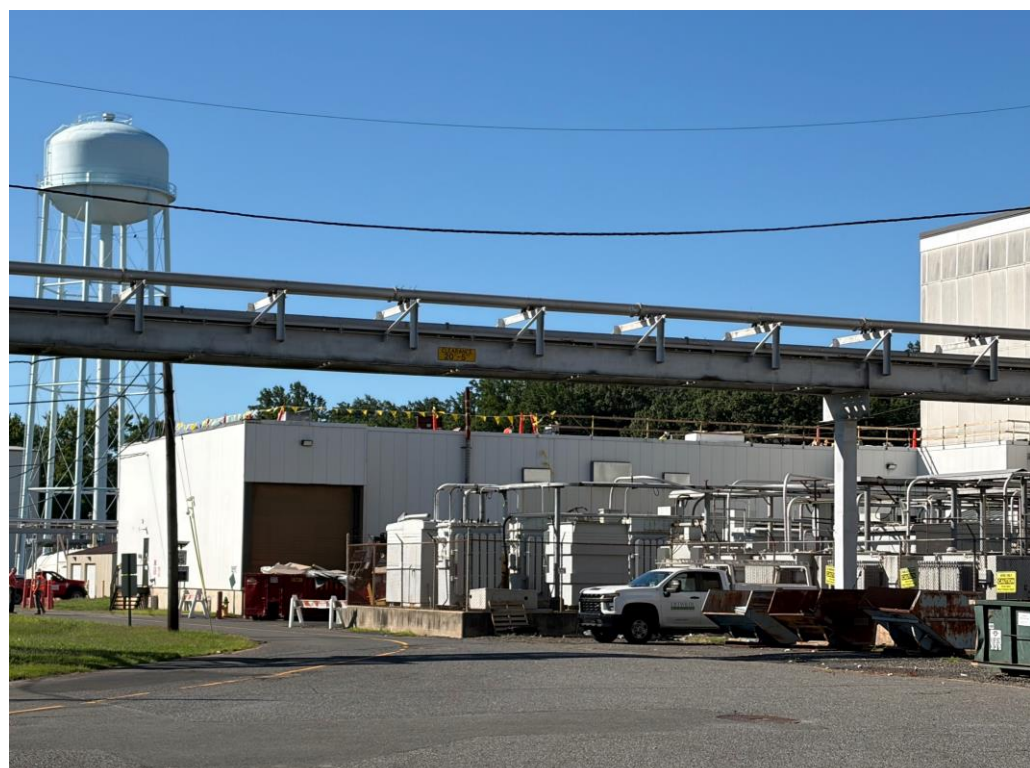
ESAT building housing LEAP Roof renovation in Sep 2026
